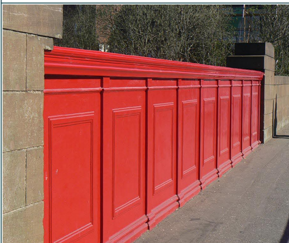
Both sides of the bridge were refurbished.
